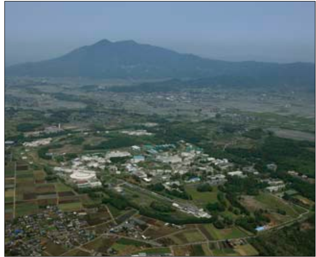
Fig. 3: Areal view of the KEK site located about 70 km from Tokyo with Mount Tsukuba in the background. The 400 m long electron/positron linear accelerator and the buildings above the collider ring whose circumference is about 3 km can be seen.
